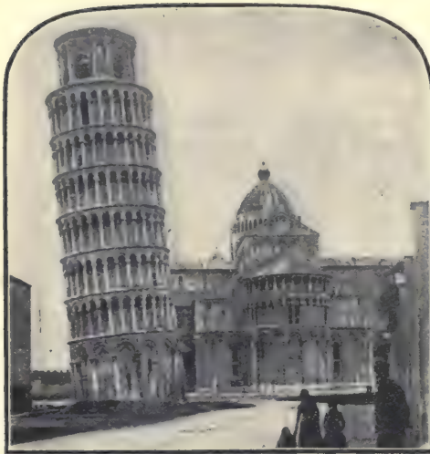
FIG. 243—Cathedral and Leaning Tower, Pisa, Italy
